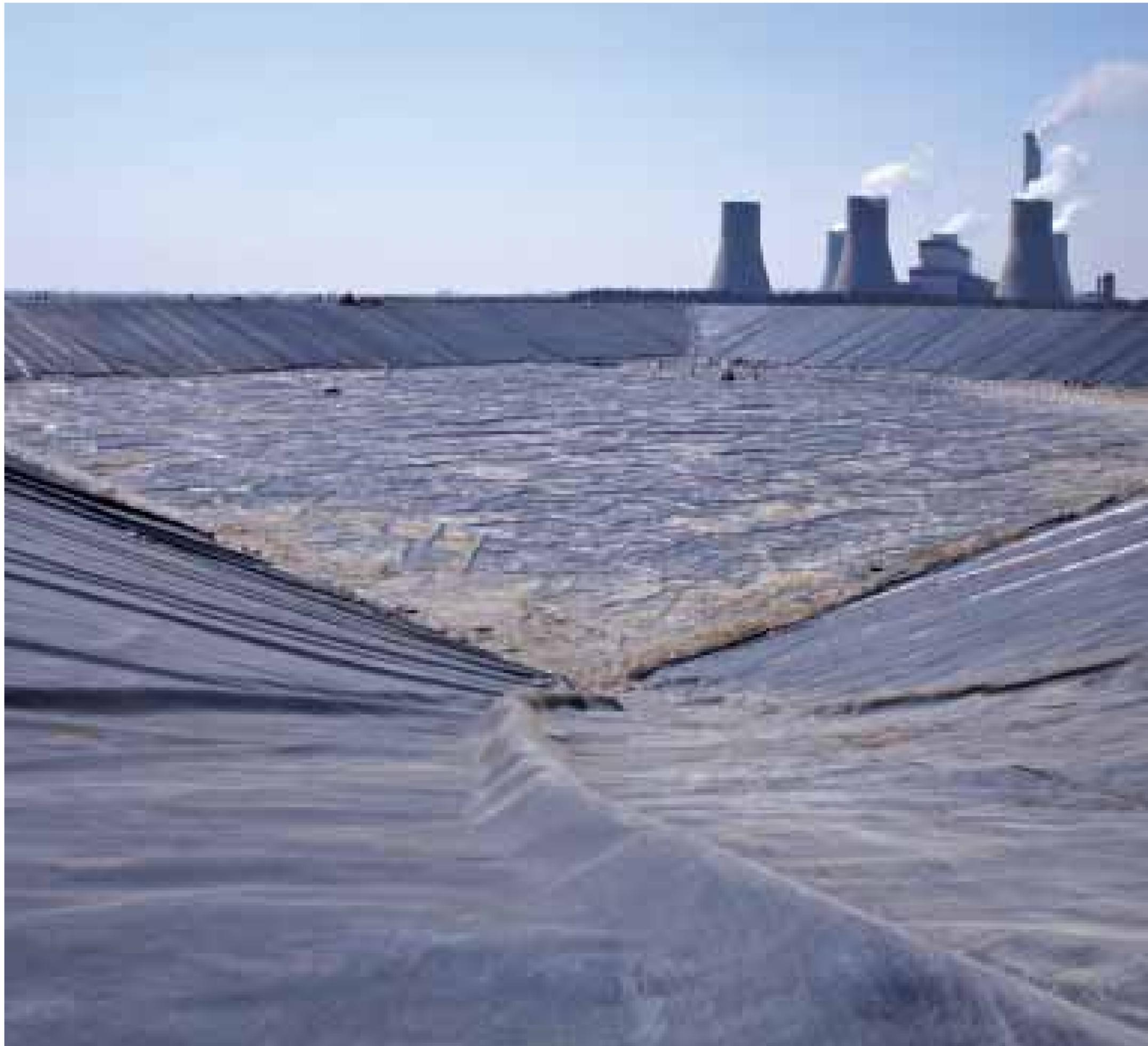
Mine Waste and MSW containment systems, especially those designed for containing hazardous materials, are lined using a dual liner system. Positioned below the primary liner and above the secondary liner is a drainage layer designed to collect leakage and often called a Leak Detection System (LDS).
