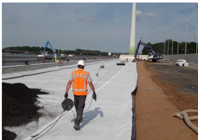
Installation was simple and required no specialist plant
