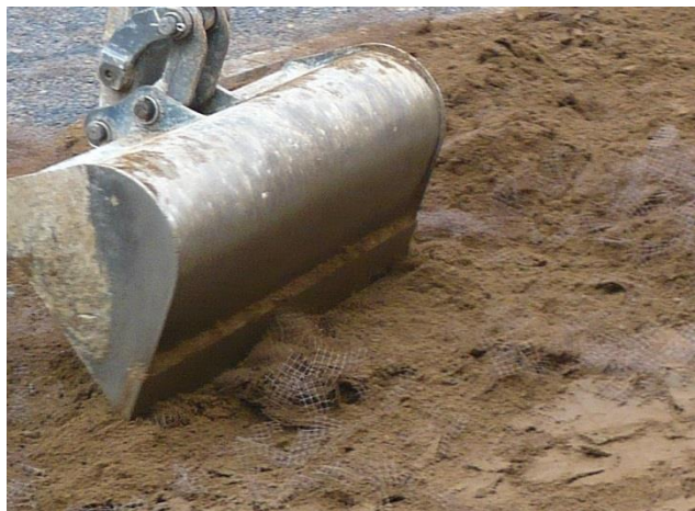
Advanced Turf System rootzone/mesh element blend (ATS400/B) being spread into access route areas
