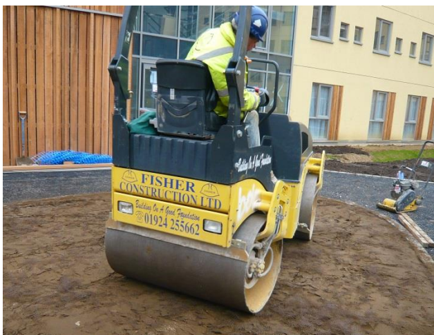
Controlled compaction of reinforced layer pre- turfing
