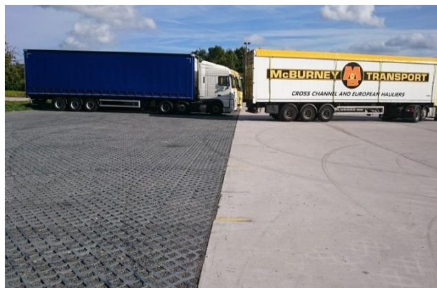
Designed for HGV braking, slewing and turning zones. Note the turning tyre marks caused by the HGVs
