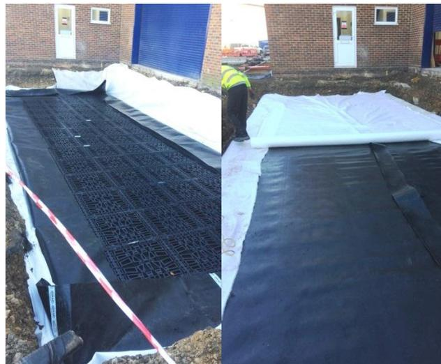
Inflow and restricted outflow pipes fitted, Alphaline LLDPE liner sealed and protected by Terrex geotextile
