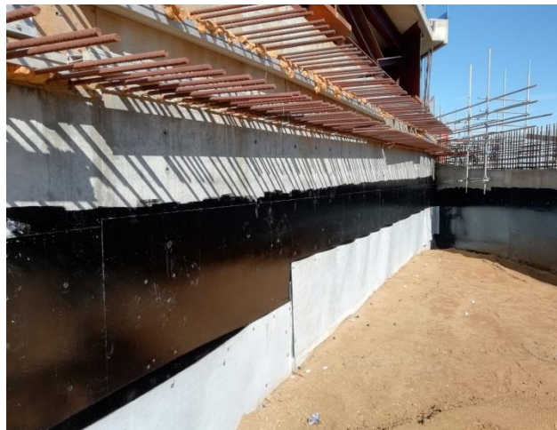
Easily and safely placed in cramped working conditions. Deckdrain provides protection to waterproofing from backfill operation
