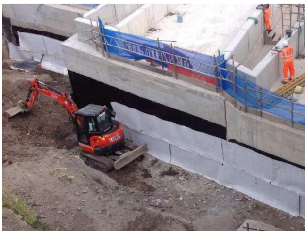
Deckdrain replaces concrete block drainage in tight work space
