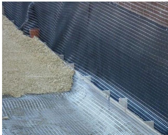
Layers of Trigrid EX30 wrapped around 500mm of crushed stone.
