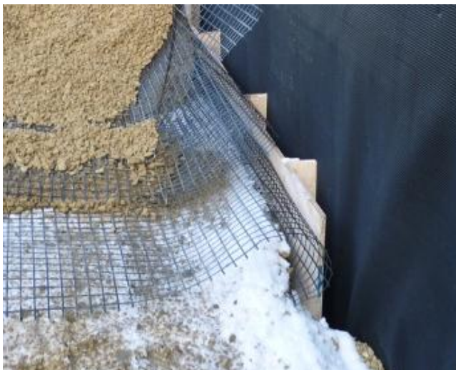
“Climbing” temporary timber void former.
