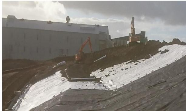
**A combination of Pozidrain with one geotextile for the flatter areas and two geotextiles for the steeper areas of the landfill capping provided significant cost savings**
