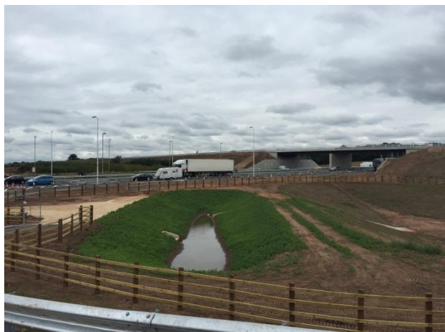
The result a protected lined balancing pond
