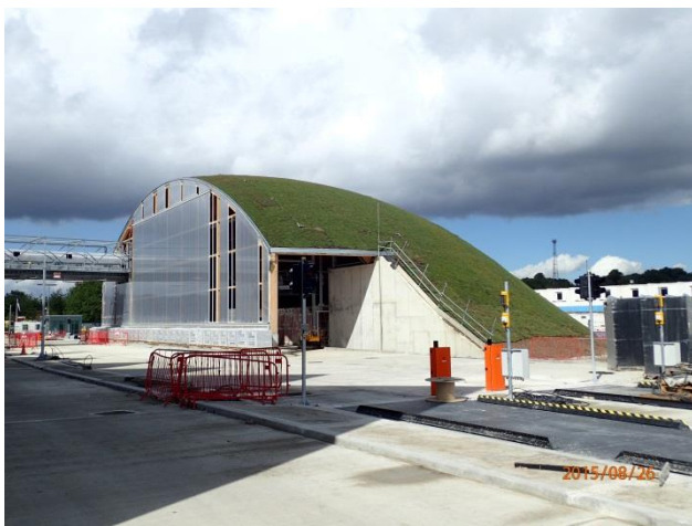
Finished lightweight ABG Green Roof System
