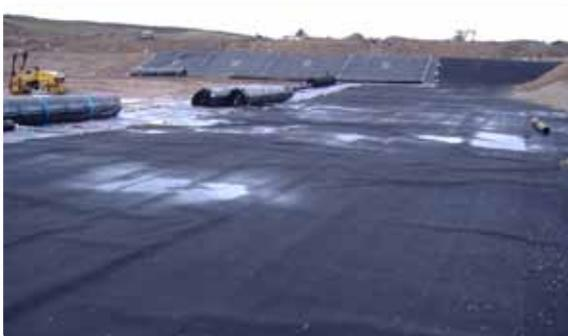
Leakdrain comprises a single cusped core with very high compressive strength performance. This high compressive strength combined with high in-plane flow capacity allows the flow of leachate and other particle laden liquids without the risk of clogging, even under very high loads.
