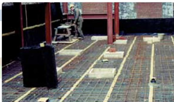
Cavidrain is a preformed cavity drainage system designed specifically to relieve water penetration from buried structures such as tunnels, basements, underground car parks. It is suitable for use in both new build and existing structures
