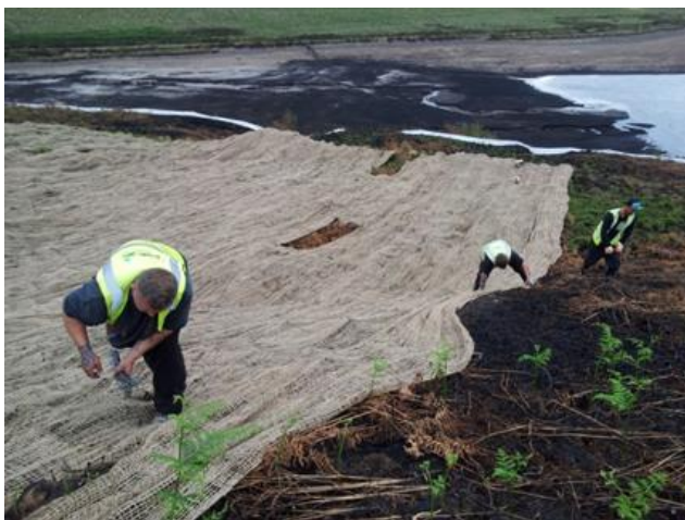
Quick deployment over burnt areas of hillside
