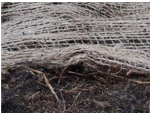
Matting pinned closely to the surface to prevent erosion
