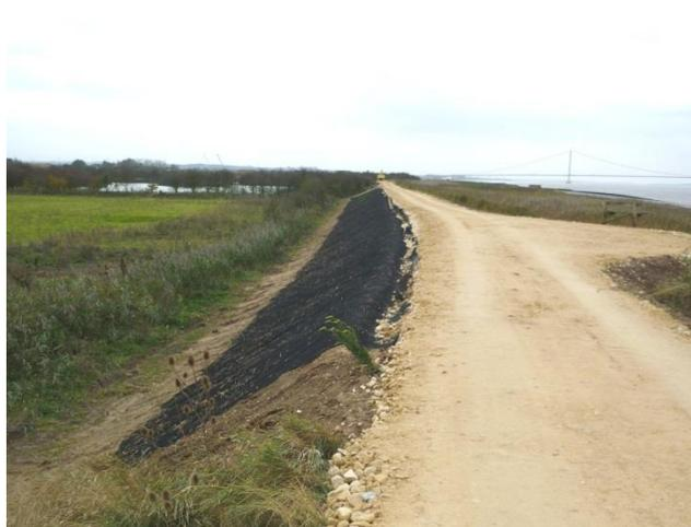
The Erosamat and anchor trench is ready for backfilled with topsoil. ABG Abgrid biaxial geogrid was used to reinforce the crest which acted as an access road.
