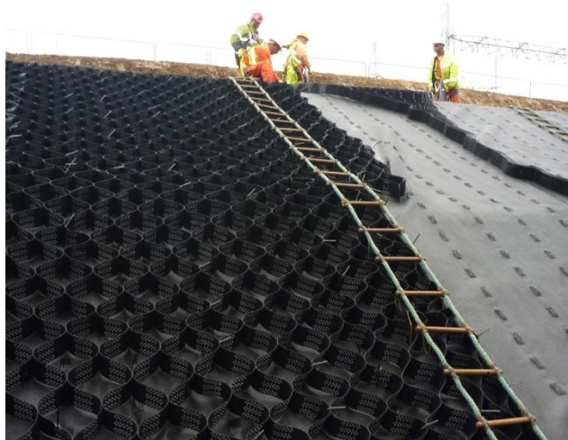
Erosaweb placed in anchor trench and expanded down slope
