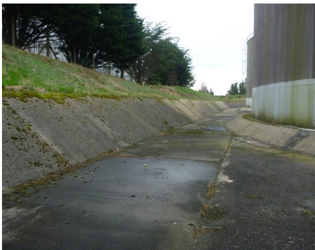
Existing bunds to be lined and extended
