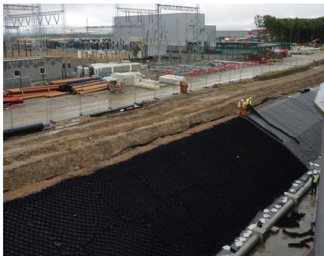
Erosaweb anchored in place ready to receive topsoil
