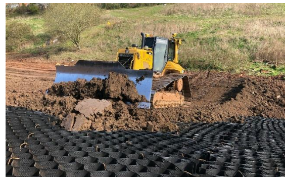
Backfilling Erosaweb panels using bladed dozer
