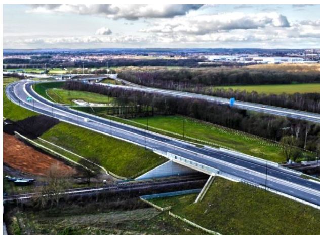
Finished stable, drained and consolidated embankment
