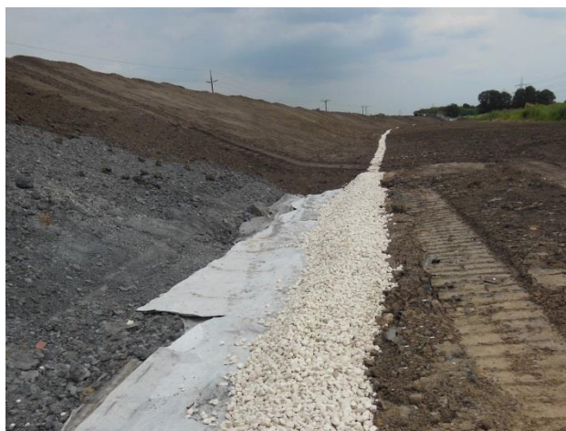
Finished embankment profile with Fildrain tucked into perimeter drain
