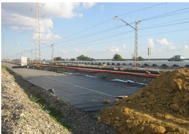
Embankment fill being installed on Pozidrain
