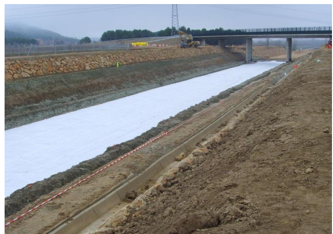
Wide width rolls allowed rapid installation to meet challenging project timescales
