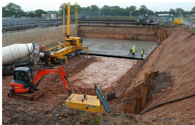
Fig 7: Deckdrain laid towards the drainage trench
