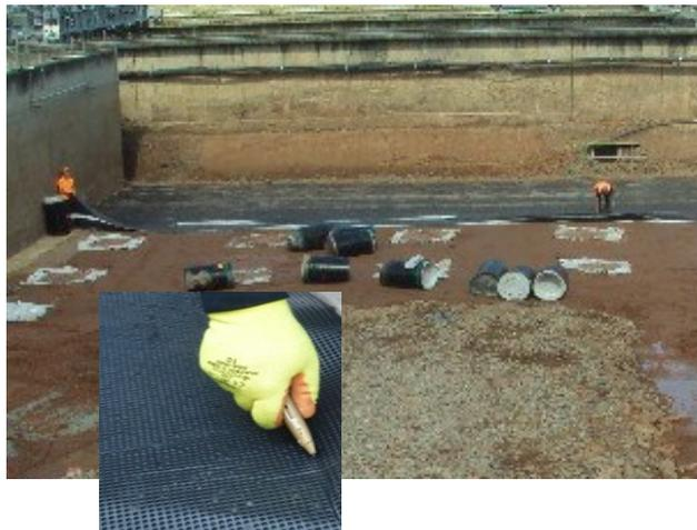
Fig 4: Rolls laid in line with direction of main flow and cut with sharp knife to suit edge details
