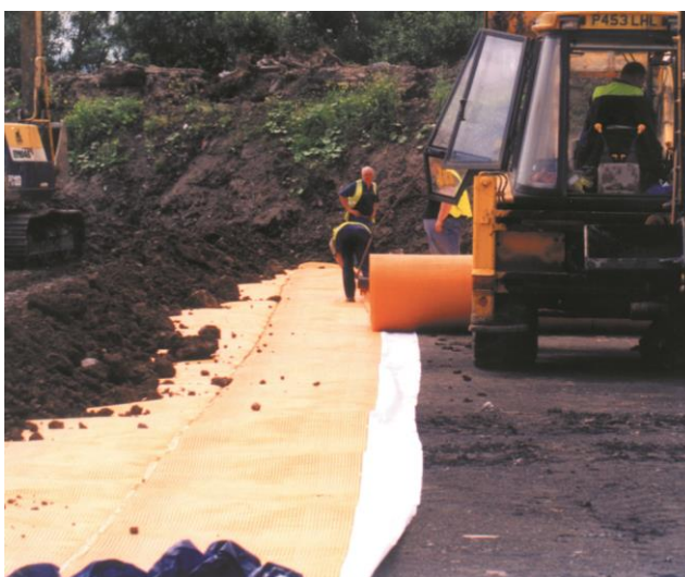
Overlapping Pozibreak rolls to form a continuous layer
