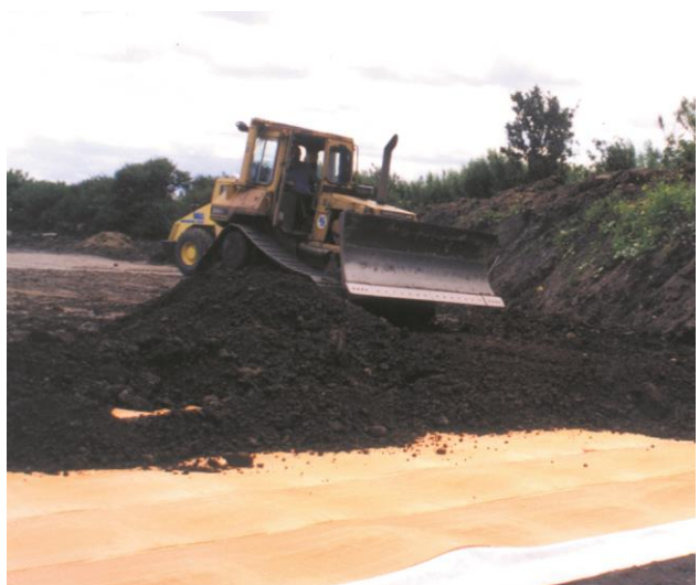
Clay layer placed on Pozibreak
