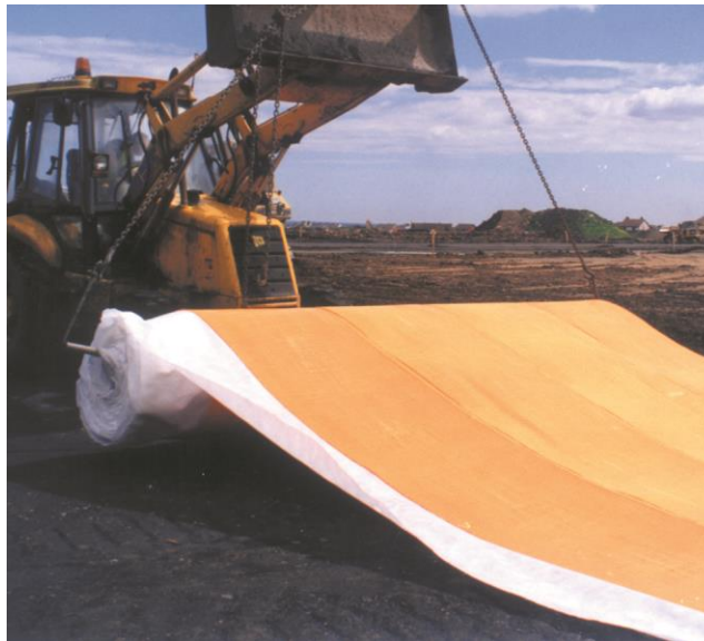
Pozibreak being installed in 4.4m wide rolls
