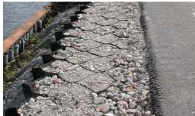
Fig. 6: Installed ConcertinaWeb Filled and compacted
