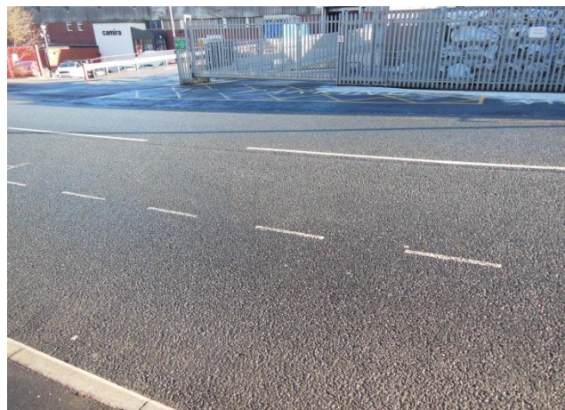
New road surface after installation late 2010
