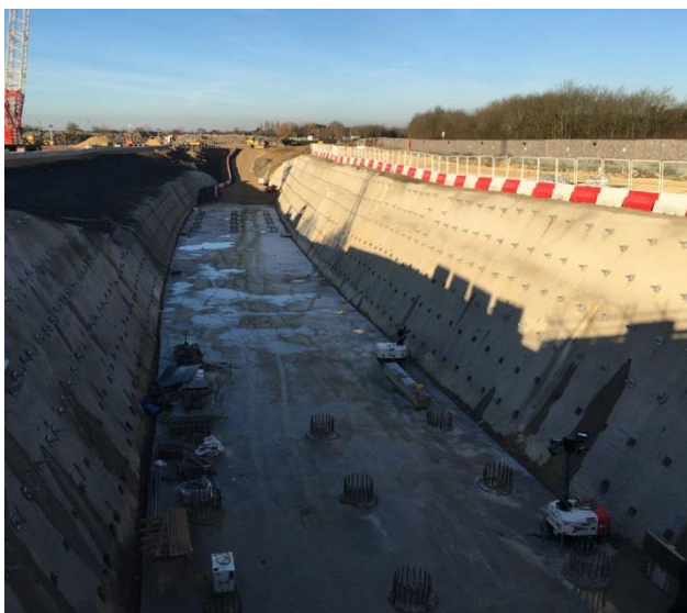
Completed retaining structure
