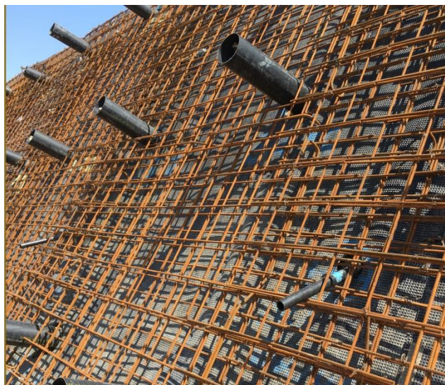
Deckdrain geocomposite, reinforcement and soil anchor installation
