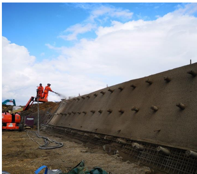
Shotcrete spraying onto Deckdrain geocomposite
