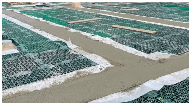
Concrete planter footings with structural drainage lining
