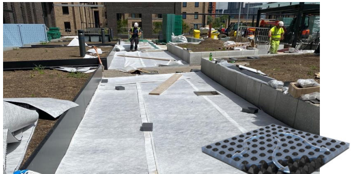
Deckdrain geocomposite layer provides filtration and multi-directional drainage performance
