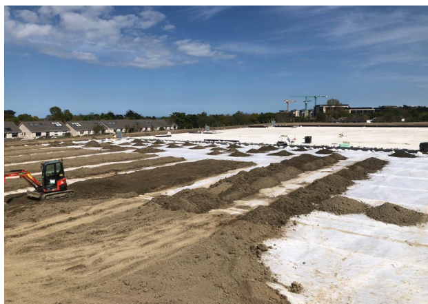
Placing of soil & growing media over the Pozidrain drainage layer.
