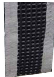
Piledrain installed to channel water from the space between contiguous bored concrete piles
