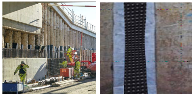
Piledrain being fixed between piles within the cutting
