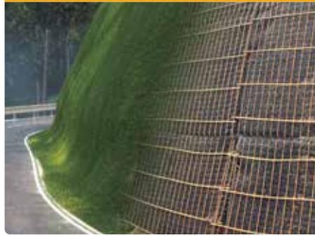
Abslope SM is an economical and structurally flexible sustainable earth retaining slope system developed for road embankments, acoustic bunds, amenity slopes, land reclamation projects and housing developments to meet the demands of Engineers, Architects and Developers. The system consists of a proprietary steel mesh facing panel and retained earth, reinforced with ABG geogrids.
