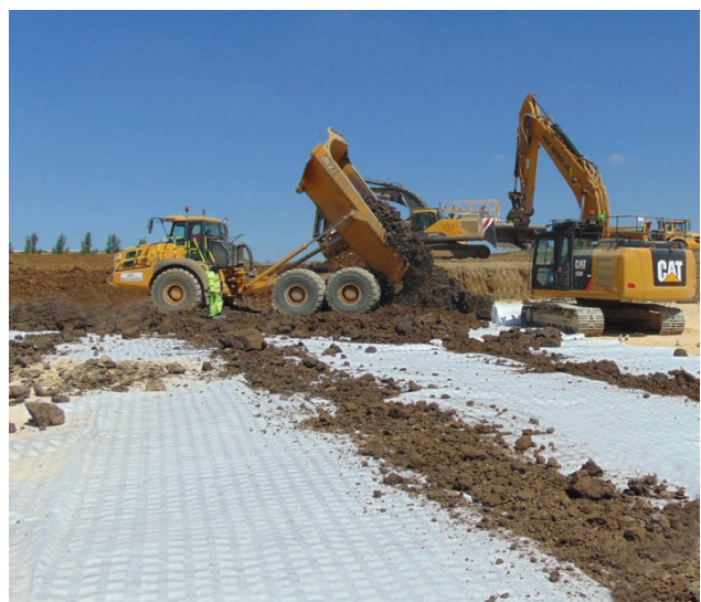
Embankment fill installation on top of Pozidrain
