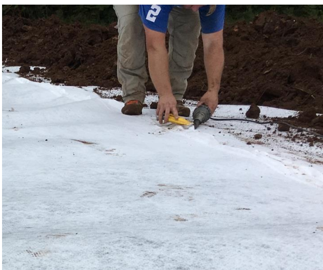
Simple heat weld joints on geotextile
