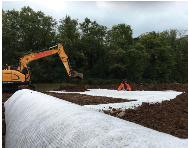
Backfill operation followed immediately behind the geotextile filter jointing
