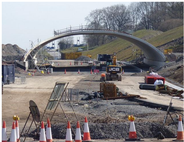
Balanced backfill operation against each abutment
