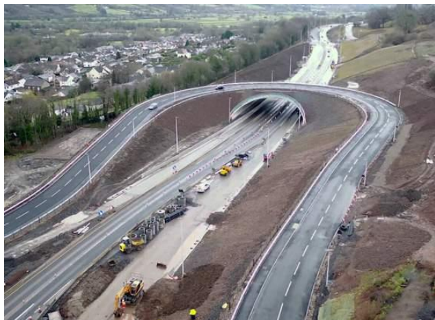
Deckdrain Contributes to the very installation of the bridge.
