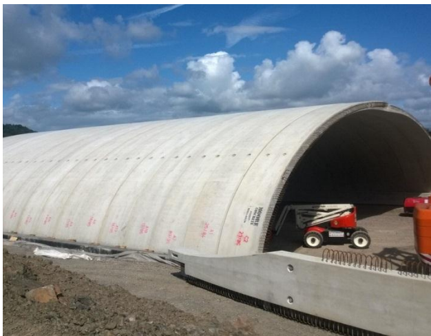
Arch units ready to receive waterproofing and Deckdrain drainage/protection geocomposite
