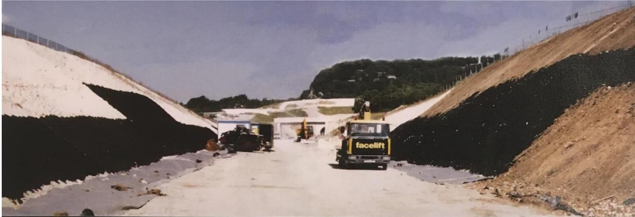
**Erosamat's** three-dimensional open matrix was utilised to protect the less steep upper slopes from erosion and to provide permanent root zone reinforcement for the vegetation. 150mm of topsoil was placed on the chalk with the 20mm thick **Erosamat** pinned on top. The topsoil was hydro seeded with a drought resistant seed mixture.
