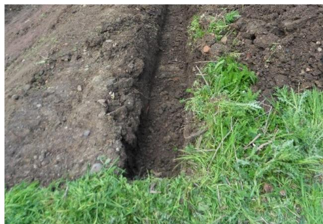
Fig 3: Excavate anchor trenches
