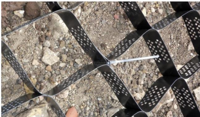
**Fig 6: Connect Erosaweb panels with Abfix Ties**
