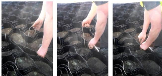
**Fig 10: Panel connection details**
