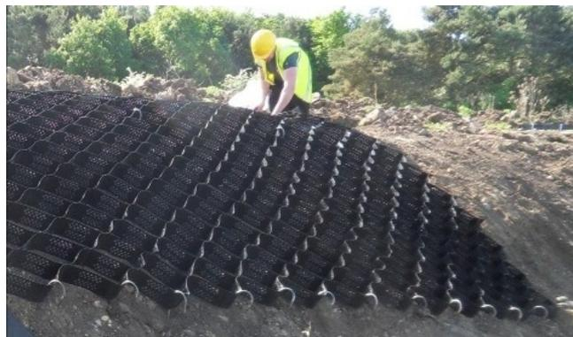
**Fig 5: Expand Erosaweb down-slope and pin in place**
