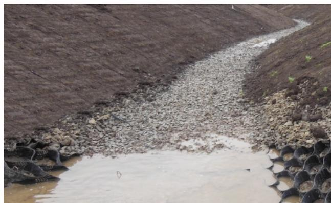
**Fig 11: Erosaweb used in a Stream Bed**
