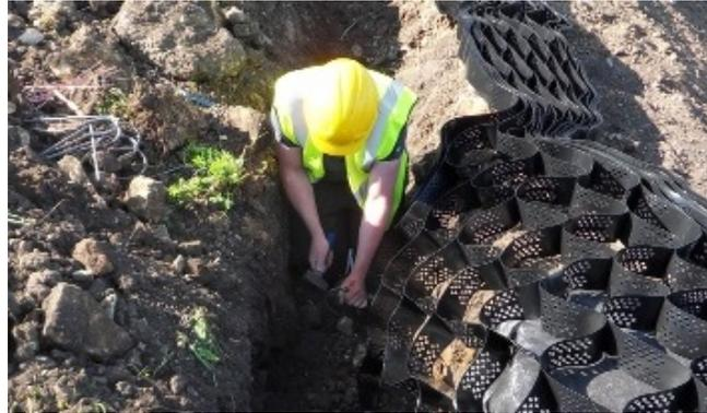
**Fig 4: Place Erosaweb and pin into anchor trench**
