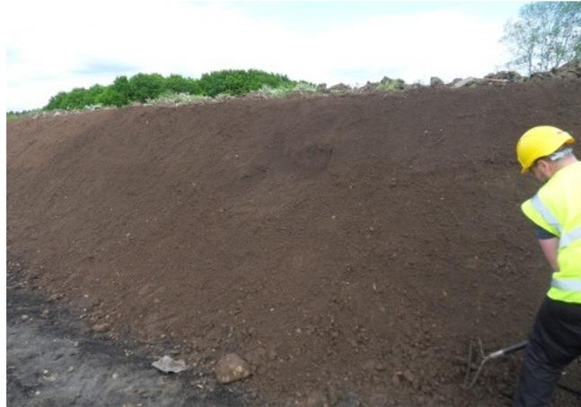
**Fig 8: Place topsoil from bottom up**
