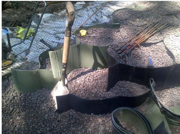
**Webwall pinned into place in layers filled with the light-weight aggregate and compacted by hand. This created a stable reinforced retaining structure supporting the road with minimal load on the embankment.**
