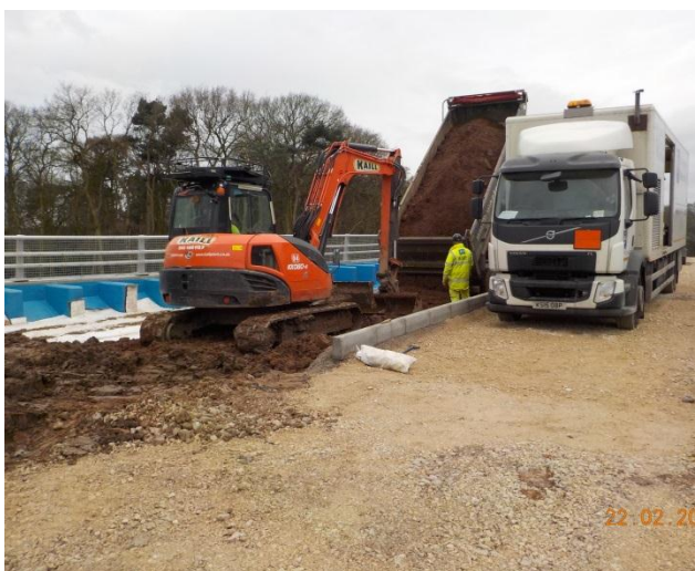
Placing of 600mm of growing media
