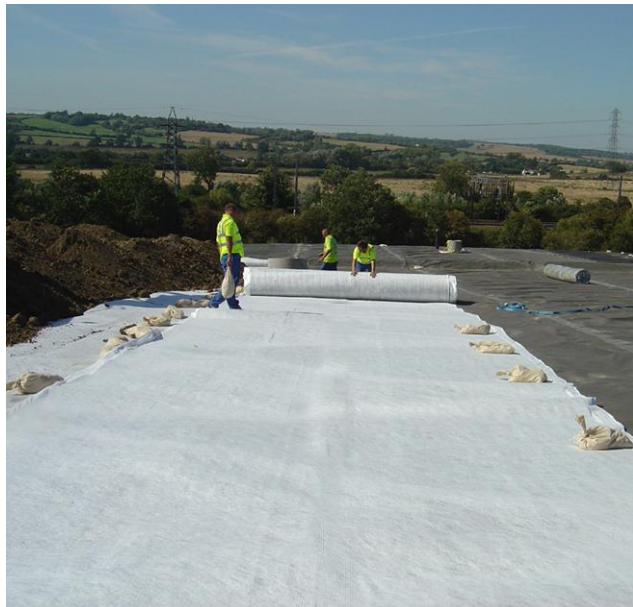
Large rolls enabled rapid installation
