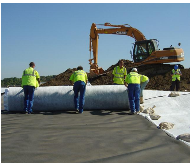
Pozidrain installed on top of 1mm LLDPE textured liner
