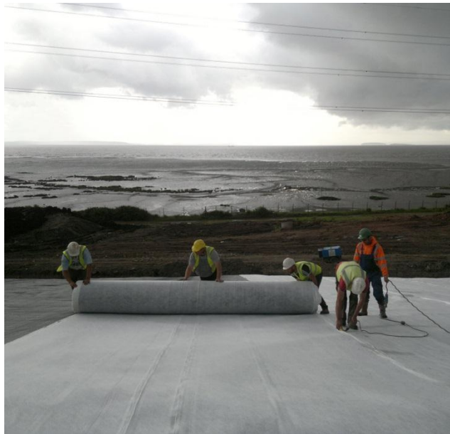
Wide-width rolls enabled rapid installation
