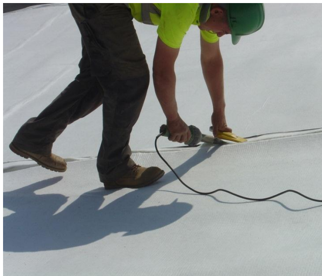
UV resistant Pozidrain geotextile tack welding with a hot air gun
