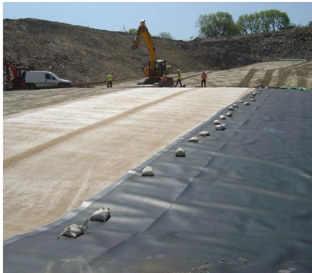
Composite lining system installation GCL and 2mm textured HDPE geomembrane
