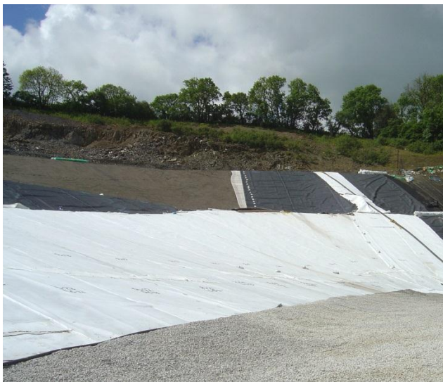
Pozidrain Protector puncture resistance ensured adequate geomembrane protection at 45m depth
