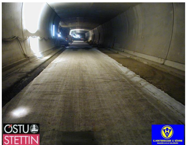
4.5m welded Deckdrain thermally bonded to Terrex Protector geotextile
