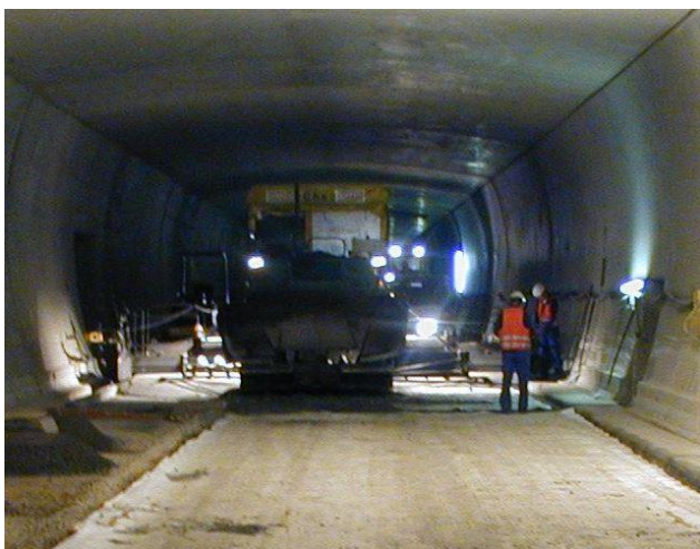
Concrete extrusion plant placing concrete onto the Deckdrain
