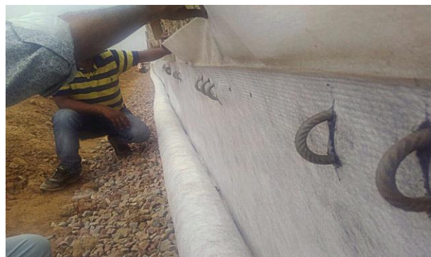
Deckdrain is easily attached to the wall with the lower end wrapped around the perforated drainage pipe.
