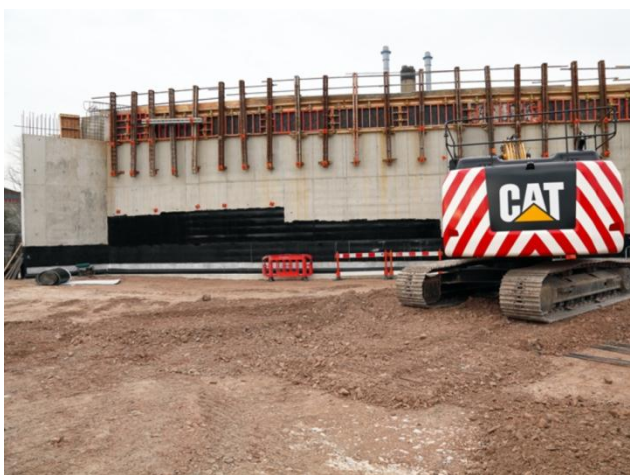
Roll of Deckdrain ready for next horizontal lift with no delay or interference with backfill operation
