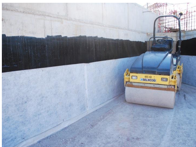
Deckdrain allows compaction close to the structure and provides protection to the waterproof coating
