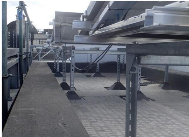
The versatile ABG Roofdrain geocomposite was fitted around footings of the PV arrays to form a continuous drainage layer
