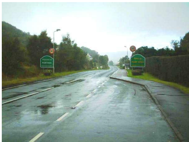
The finished road surface handling the weather
