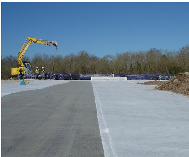
Claymat GCL installed between Pozidrain geocomposites
