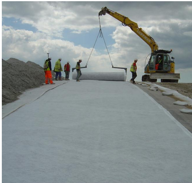
Large Pozidrain rolls enabled rapid installation
