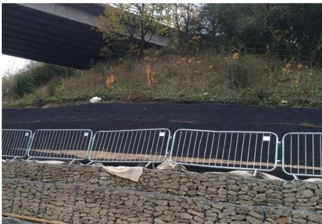
Erosamat 3/20Z 500M ready to receive topsoil and seed
