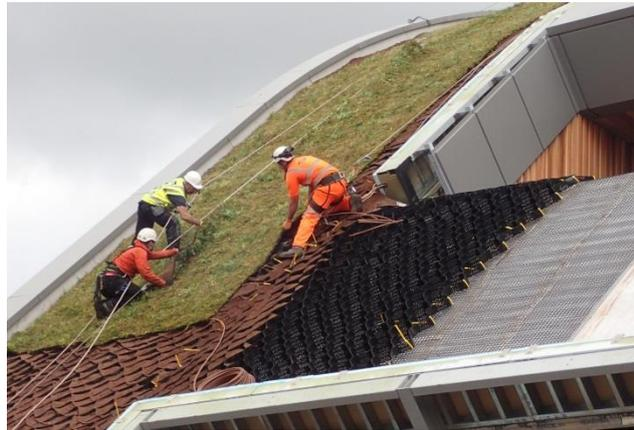
**Installation of the geocellular system (Erosaweb) to retain growing media on slopes. All Geogreen operatives were Irata level 3 & 4 trained as rope access was critical.**
