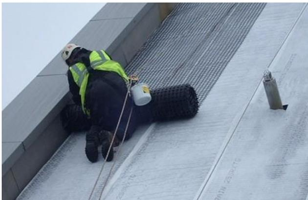
**Reinforcement geogrid (Trigrid) secured to anchor points installed above the reservoir & drainage layer (Roofdrain).**
