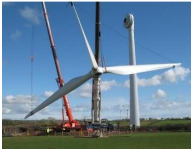
Truckcell provides a stable working surface for cranes to operate
