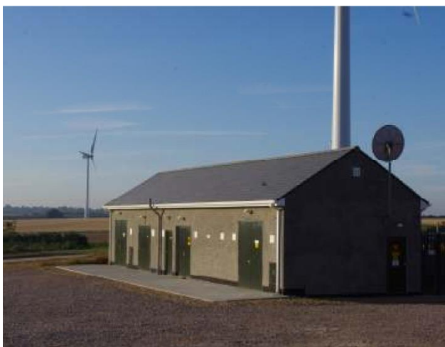
Hardstandings with blended "soft" looking edge detail
