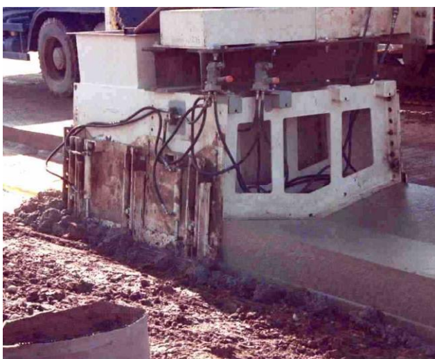
Channel extruded directly onto ABG Fildrain Type 10
