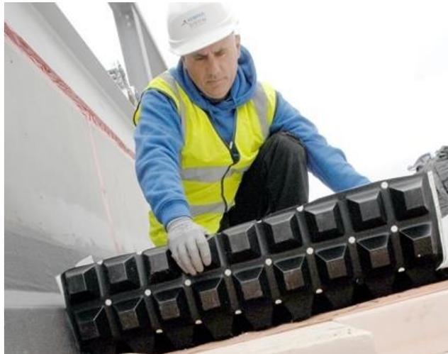
Placing the ABG green roof boards showing the overflow holes which then feed into the bluroof attenuation system below
